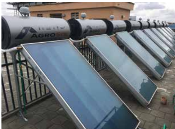
150L Thermosiphon system installation in Nairobi, 2016
